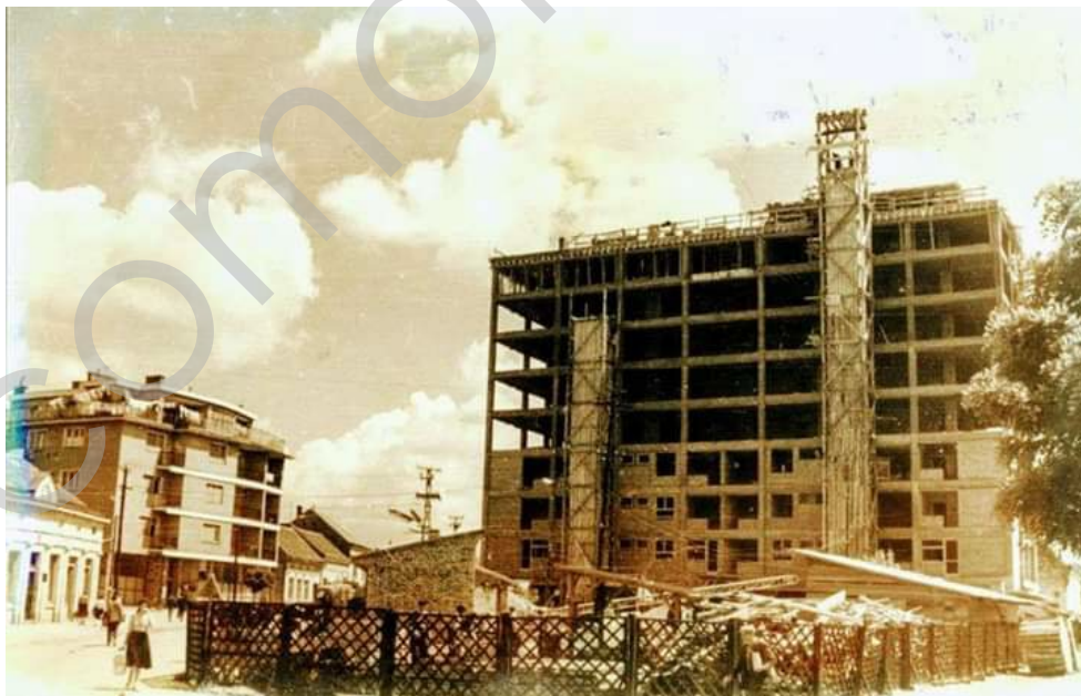
Zorka's high-rise during construction (Photo: National Museum Šabac)
